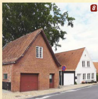
Bodhuse, mod baggade
