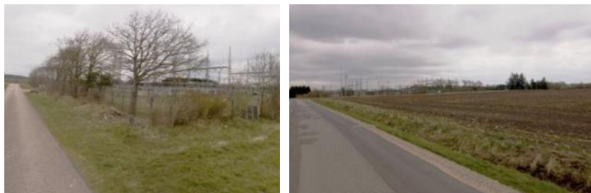
Figur 6. Bredebros Energinet Station beliggende langs Galgemark.
