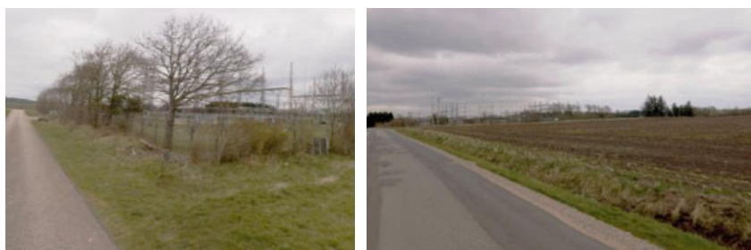
Figur 6. Bredebros Energinet Station beliggende langs Galgemark.
